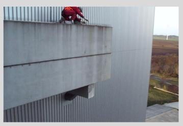
concrete patching & crack pressing of external facade and silo foundations • pressing, gelling
